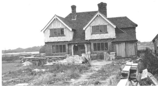
Some of the early houses being built in Kingswood
